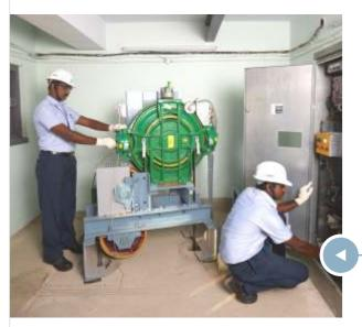
nergy savings is an important factor of the Modernization. KONE's highly eco-efficient EcoDisc® powers the elevator and as the elevator is in constant use, KONE has installed a regenerative drive that recovers upto 50% of the energy consumed.
